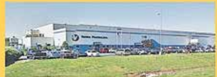
VENTRA PLASTICS Various Building Expansions & Alterations
