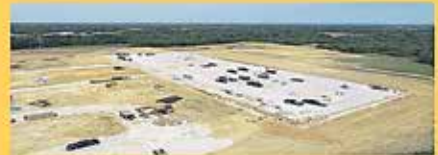
SCHUPAN & SON INC. New Aluminum Processing Facility
