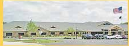
CREEKWOOD NURSING & REHAB CENTER Concrete Construction
