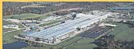
LOGAN ALUMINUM Various Expansions, Renovations & Maintenance Projects
